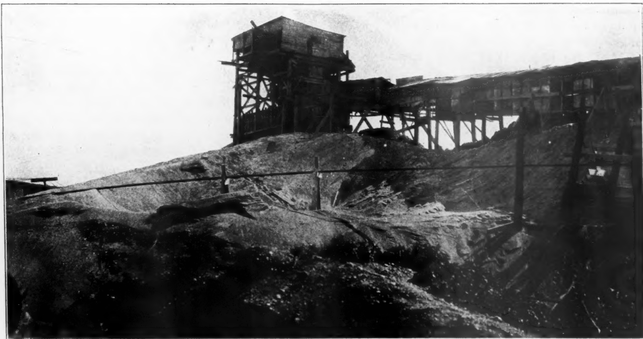
Another View of the Sand Storage and the Crushing and Screening Plant
